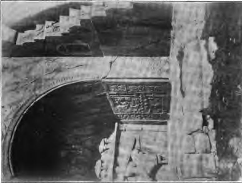
VIEW OF THE LARGER ARCH
